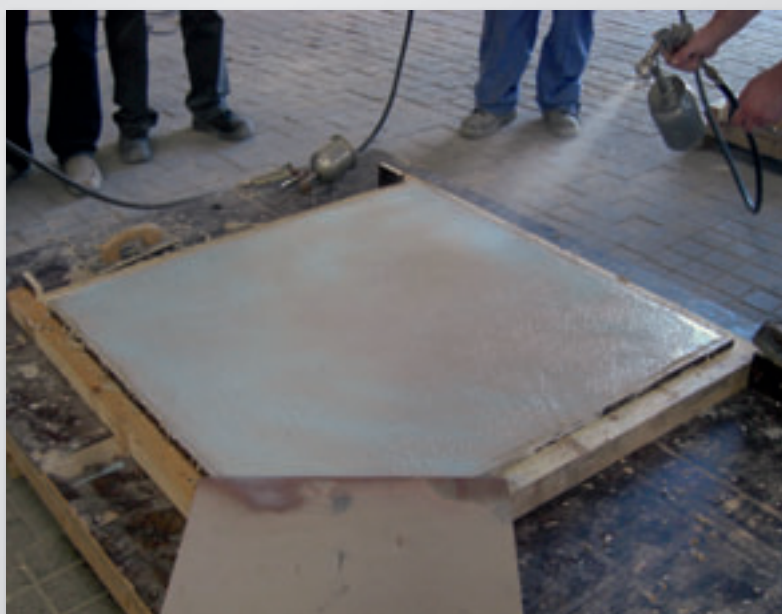
apply the retarder on fresh concrete
